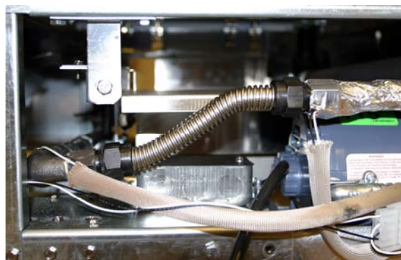
Figure 1: The flexline is behind a panel on right side of the lower back panel.
