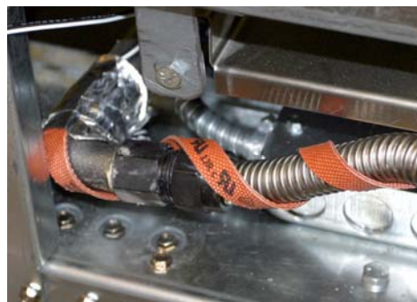
Figure 2: The heater tape is wrapped around the flexline and fittings. NOTE: Take care NOT to OVERLAP the heater tape on itself or another heater tape.
